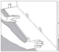
Step 1: Begin installation working from left to right. Insert spacers at ends and edges where planks meet wall to maintain 1/4" expansion space
